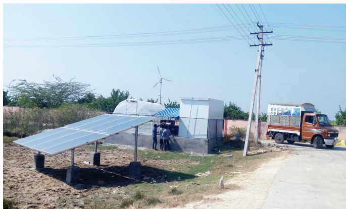
Hybrid Solar-Wind Powered Chilling Chamber and Dehydrator installed at the Fishing Harbour in Machilipatnam, Krishna District, Andhra Pradesh.
